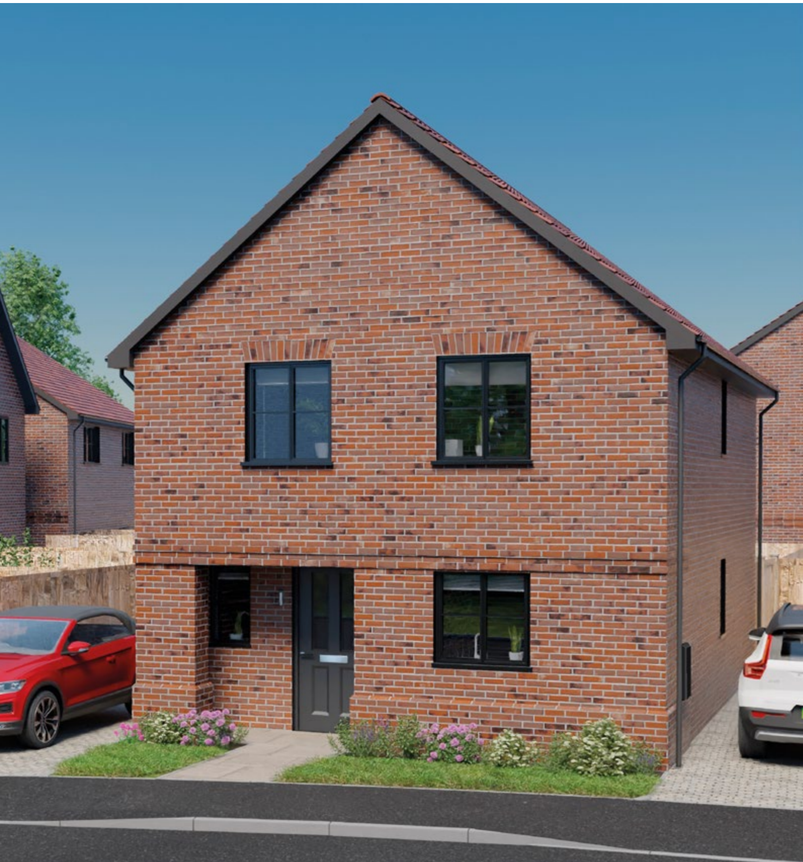
Exterior finishes may vary, speak to the sales team for more information. Computer generated image of plot 71 The Babingley is indicative only.
