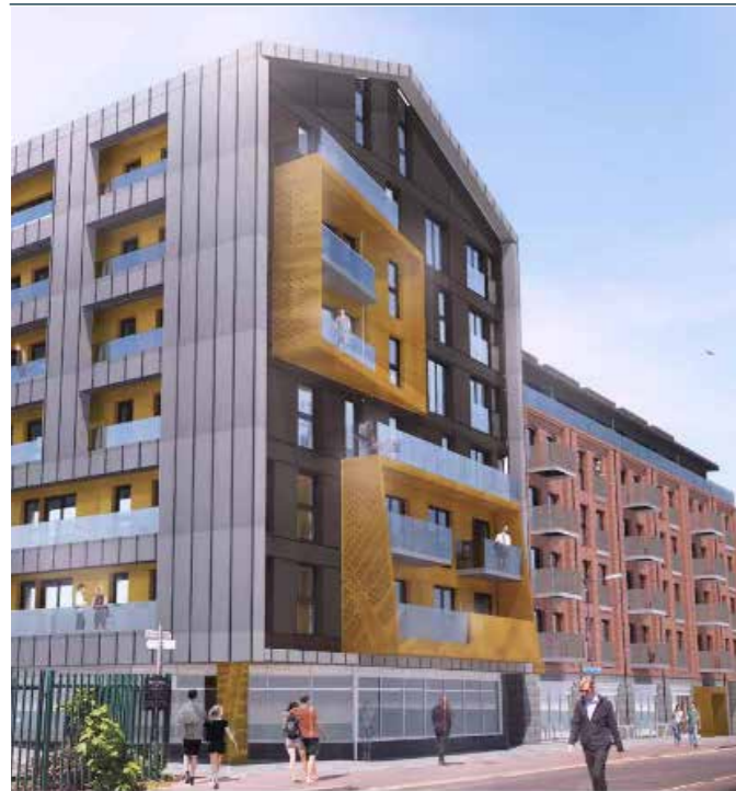
MCARTHUR'S YARD Bristol Partnership with Guinness Homes 142 homes; 1608 sq m commercial space Under construction
